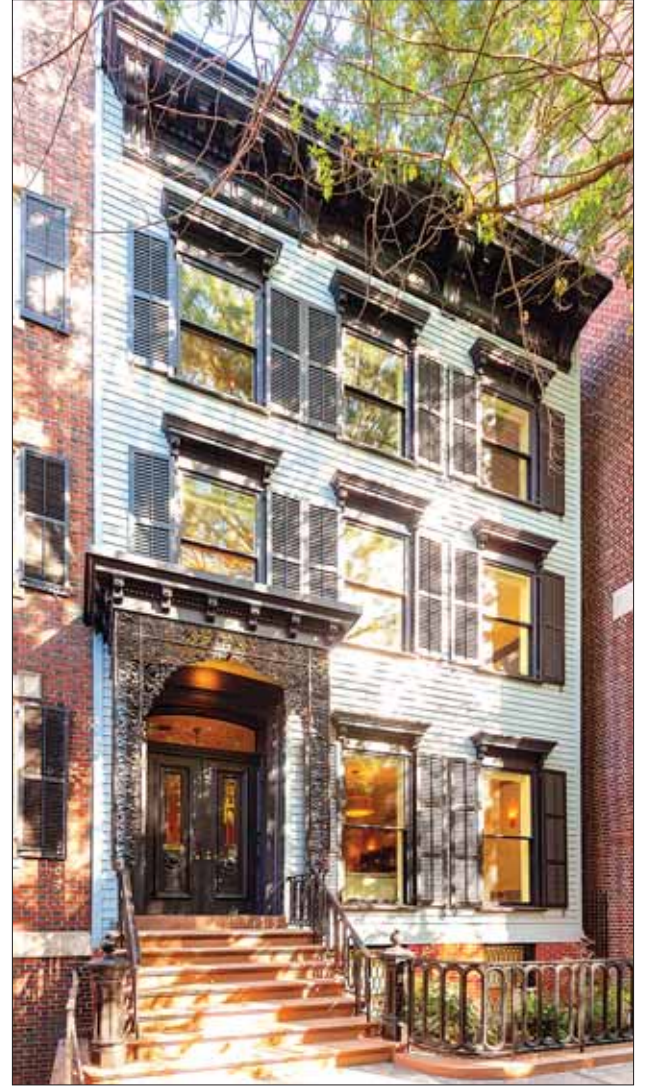
The exterior of 113 Willow St.
